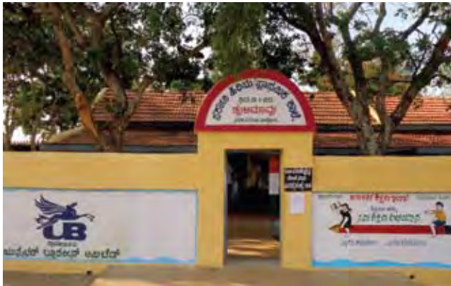
Primary school refurbished in Nanjangud, Karnataka.
